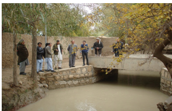
“ FIGURE 01: Construction of a culvert in Chamtal, Balkh ”
