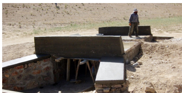
“ FIGURE 08: Culvert constructed in Tagha-e Temore village, Ghor ”
