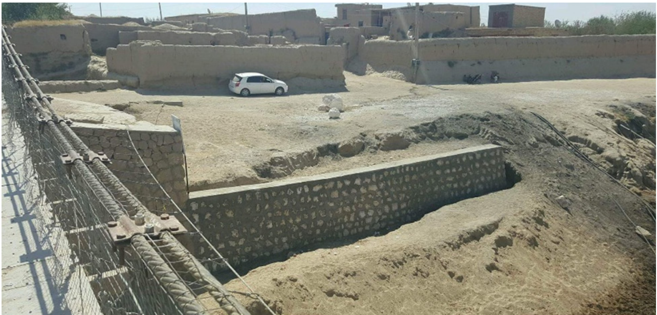
FIGURE 05: Construction of culvert, Charshangtue village, Faryab
